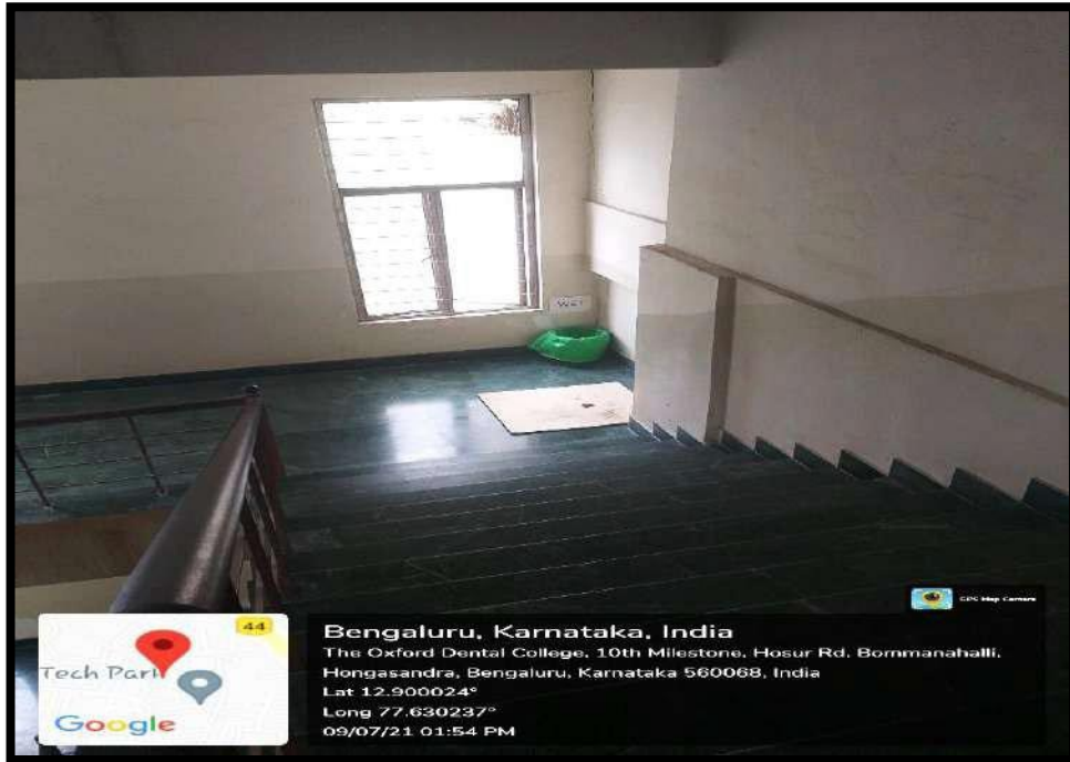
Dustbin in second floor Staircase
